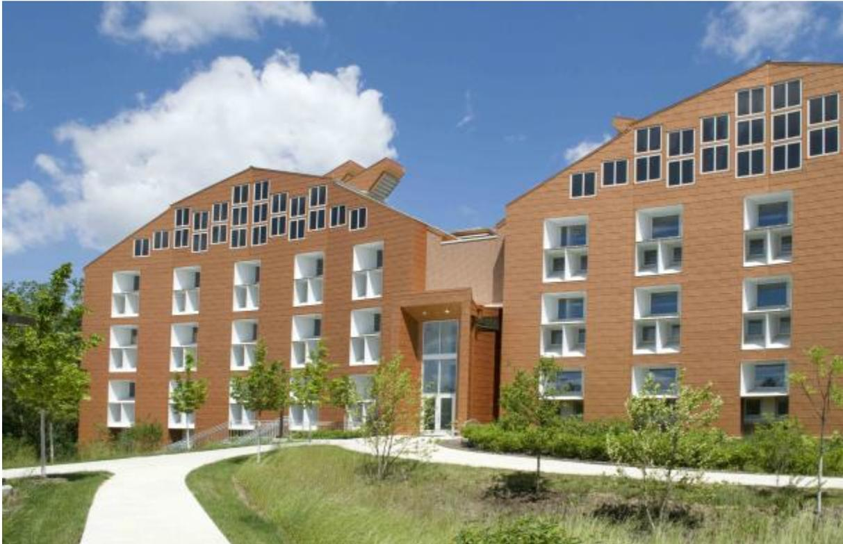
In addition to the cool metal roof, other sustainability features of the new building include exterior walls that sit four feet from the concrete structure to utilize the natural tendency of warm air to rise, creating a vacuum that draws cool air in from the bottom, circulates it and exhausts it through rooftop ventilators.
